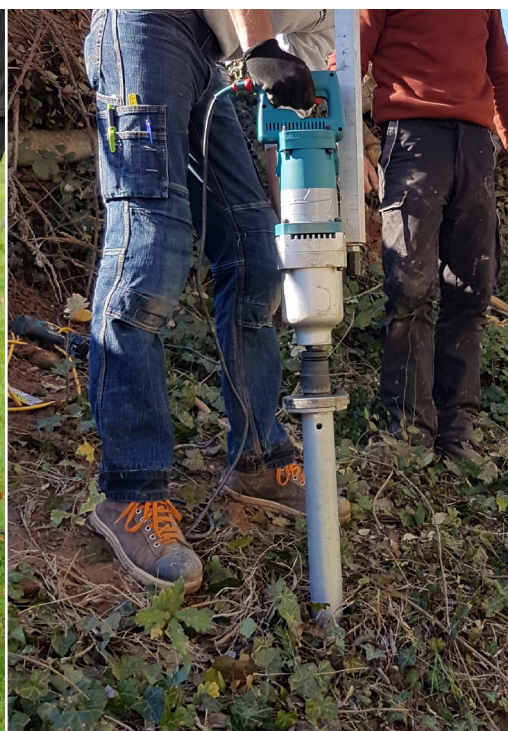
Weasylelectric Pro impact driver for installing foundation screws.
