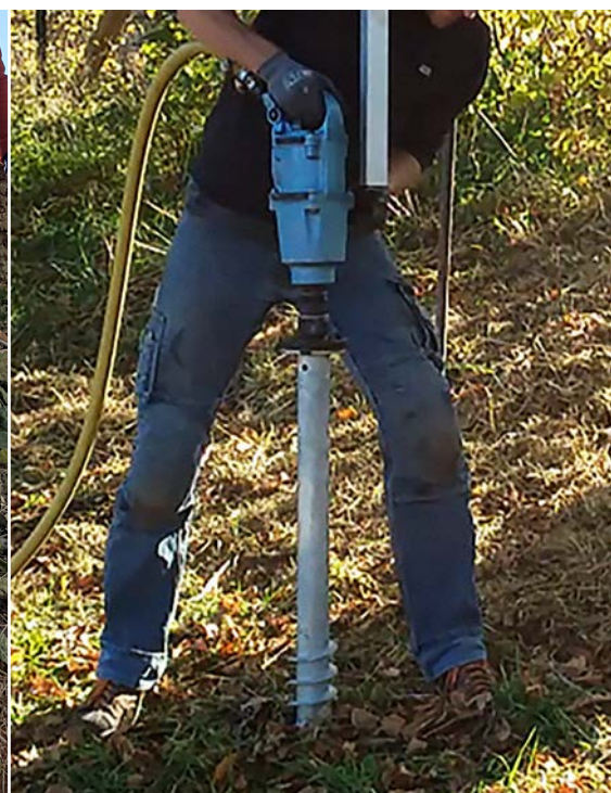
TOKU MI-4500 ESR impact driver for installing foundation screws.
