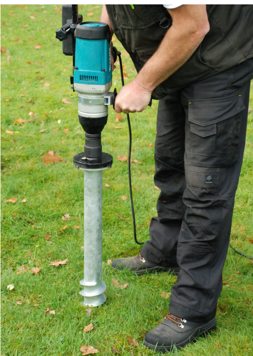
Makita TW 1000 & Hikoki WR25SE WAZ impact driver for installing foundation screws.
